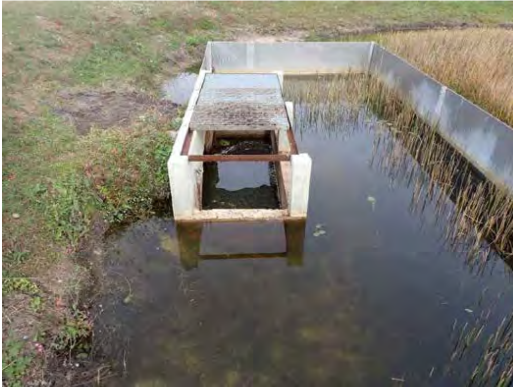
Missing Grate on Control Structure at Pond 4C
