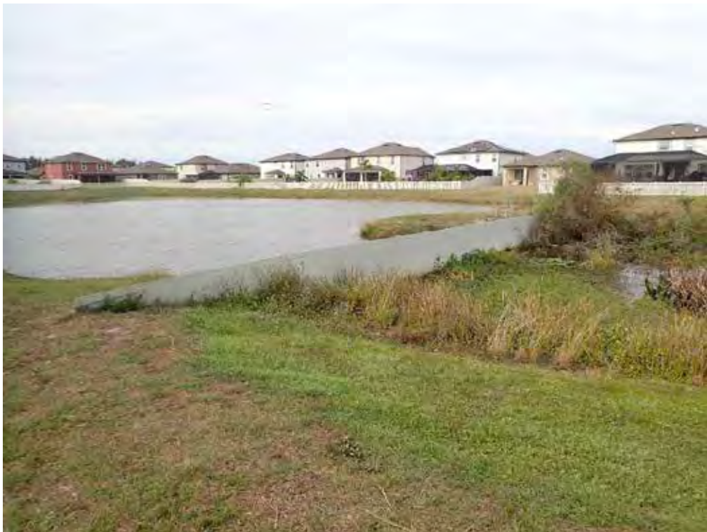
Skimmer and Weir between Pond 4B and WCA B. Vegetation needs removed from this side of the skimmer and from adjacent to the submerged weir wall
