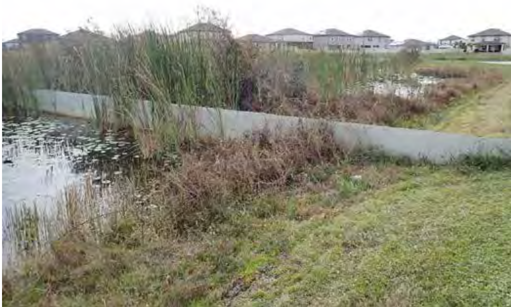
Skimmer on NE corner of WCA -B adjacent to sediment sump. Vegetation should be maintained to keep clearance from the skimmer to minimize opportunity for blockages.
