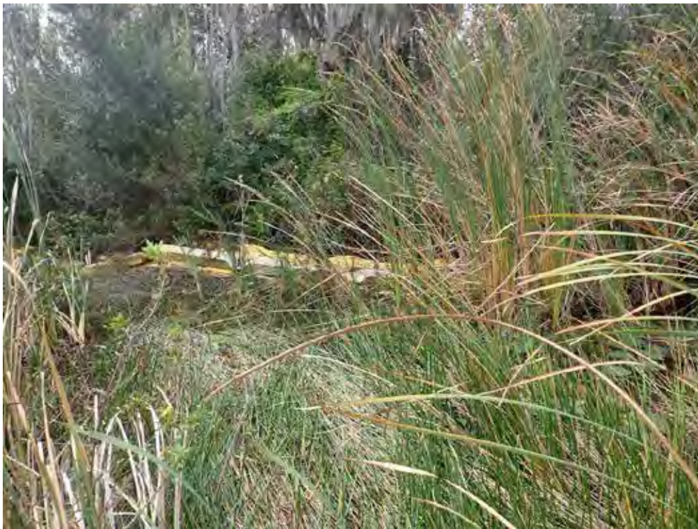
Floating turbidity barrier in place to minimize turbid discharges during home construction should be removed and disposed.
