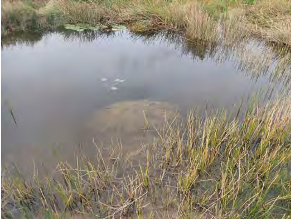
Exposed pipe end on Pond 4A; Flared End Section (FES) may have eroded into pond
